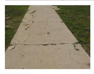
System: G2020 - Pedestrian Paving - sidewalks, etc
